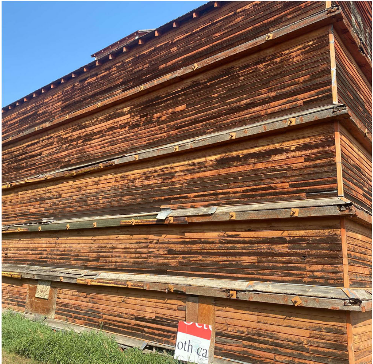
Figure 3: Structure Steel View from Exterior
