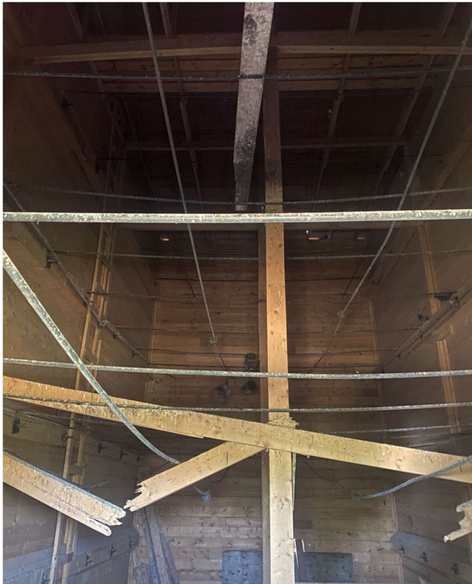
Figure 2: Structure Steel Supports
